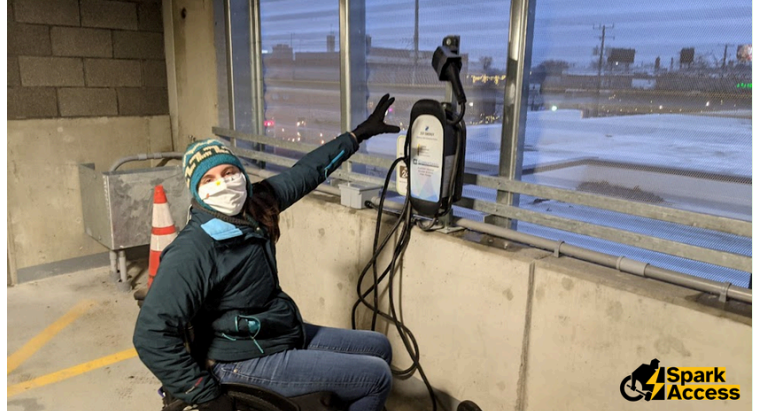
A woman using a wheelchair attempting to reach an L2 charger that is beyond 48"
