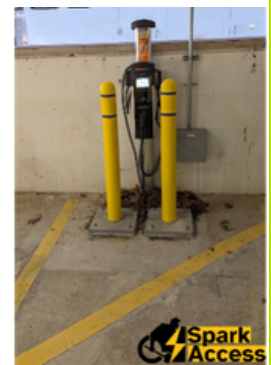
Bollards overused to impede Barrier-free approach and clear floor & ground space for EV Charger, Ann Arbor, MI
