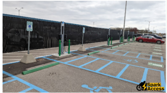
Example of van accessible EV charging spaces. Flo site in Warren, MI
