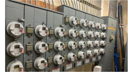
Unit electric meters in Cascadian Court electrical room
