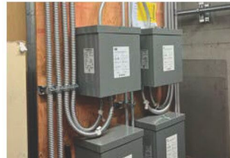
The EVEMS system in Cascadian Court's electrical room
