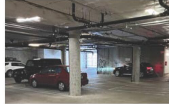
Cascadian Court Parking Garage
