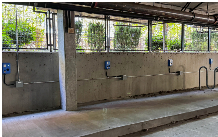
Pando Smart Level 2 Outlet daisy chain at a Woodland Creek Condominium parking garage
