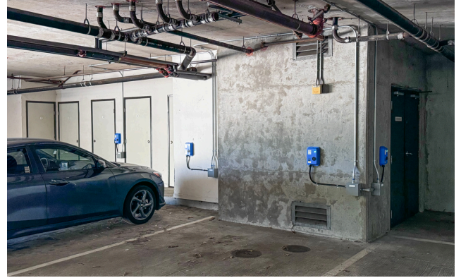
Pando Smart Level 2 Outlets in one of the Woodland Creek Condominium parking garages
