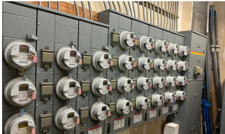
Unit electric meters in Cascadian Court electrical room
