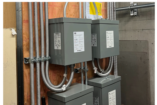
The EVEMS system in Cascadian Court's electrical room
